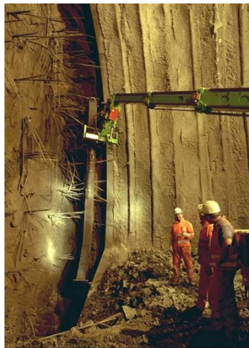
Fig.3 Centine e spritz-beton
